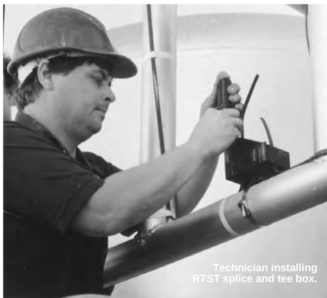
OMEGALUX® heat cable shown installed on piping and valves. Heating cable is held in place by FT-2 fiberglass tape.
